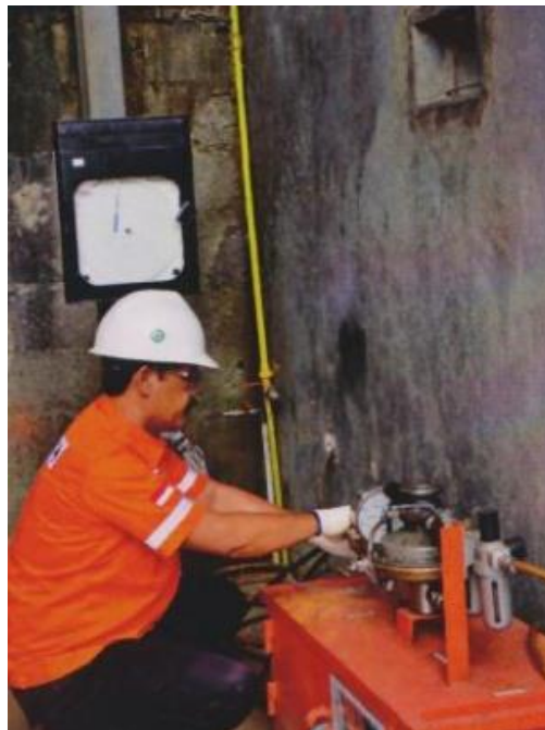
Gambar 4.8 Mesin Hydrotesting (Sumber : PT Bima Drilling Tools)
