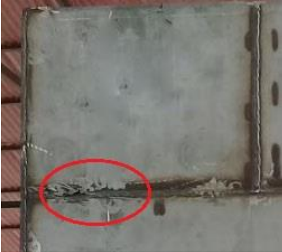
Gambar Cacat Incomplete Penetration
