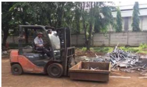
Gambar 4.16 Proses Pindahan Material
