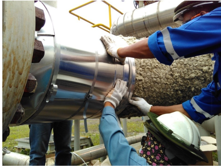
Gambar 4.4 Proses Pemasangan Aluminium with Polykraft Moisture Barrier
