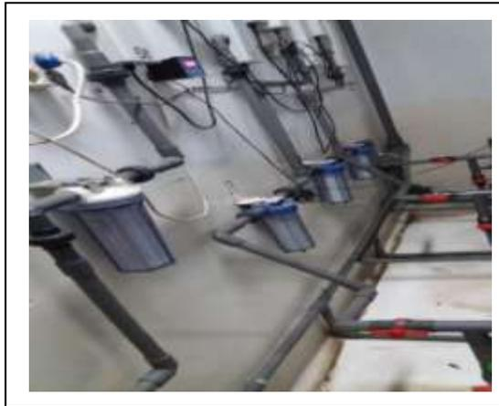
***Gambar 4.14 mesin Filter/catridge***
